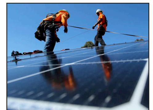
Solar installers place solar panels on the roof of a residential home in San Diego on Oct. 14, 2016. Photo by Mike Blake, Reuters
